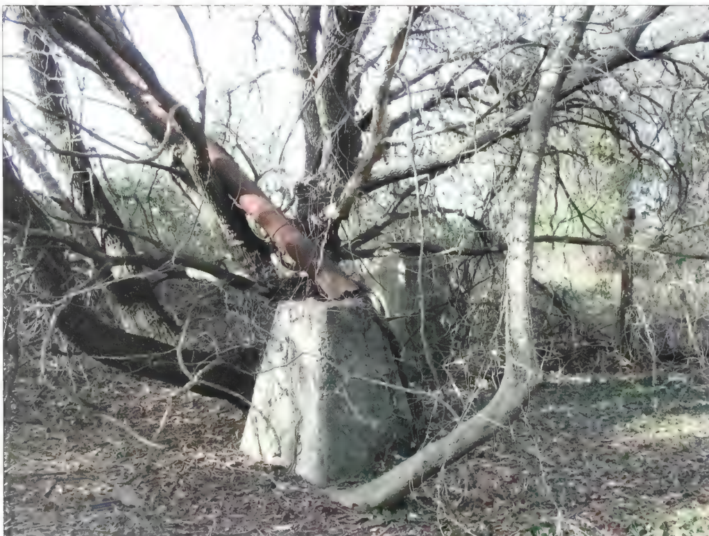
Figure 3.52. View looking northwest from the top of Battery Mills. A tapered concrete box and metal pipe are located near the center top of the engineered earthwork. These structures are most likely associated with ventilation or served as flues for furnaces (Olmsted Center, January 2009).
